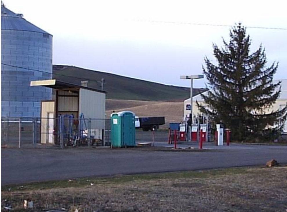
Bulk fuel distribution
