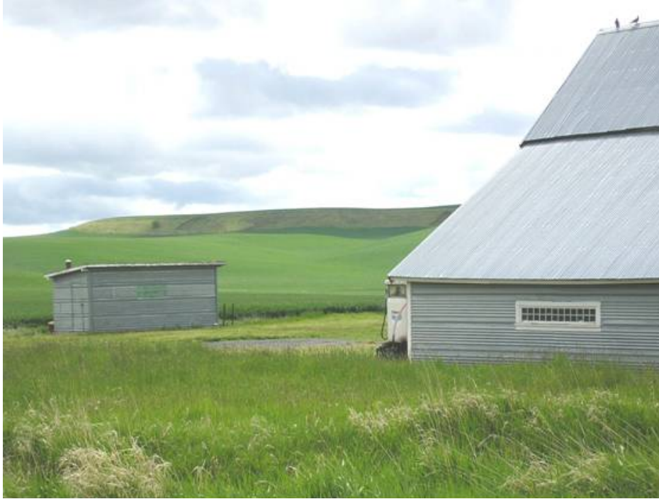
Typical fuel pump (UST)
