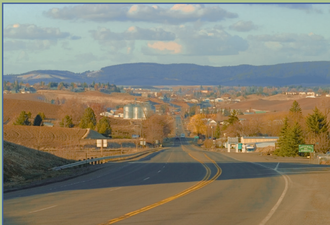
The U.S. 95 Thorncreek Road to Moscow Project is a study to determine an alignment for nearly 6.5 miles of U.S. 95 in Latah County.
